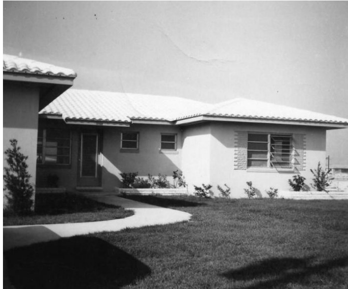
House at 11160 Sixth St E, Treasure Island, near St Petersburg, FL
