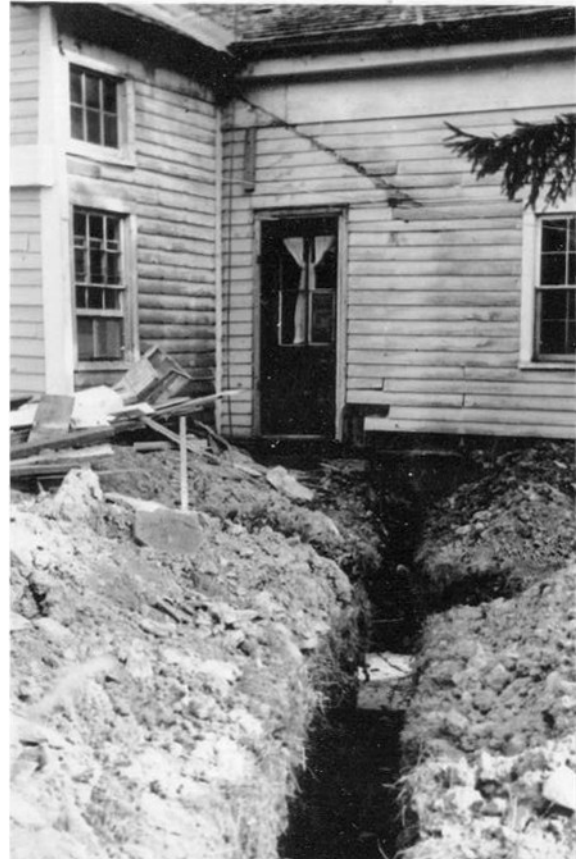
Trench from house for sewage pipe
