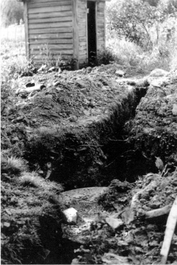
Septic tank in position
