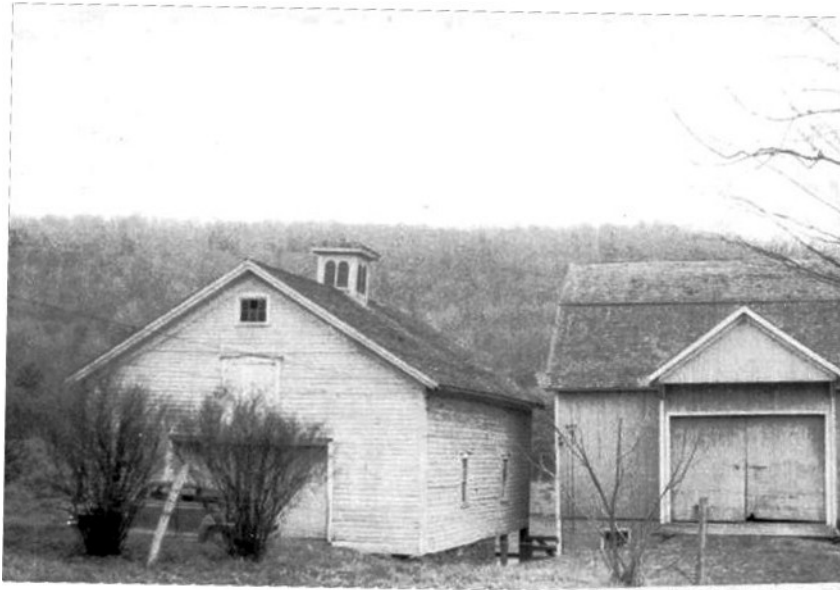
Across Bundy Hollow Road from house: Barn and other outbuilding
